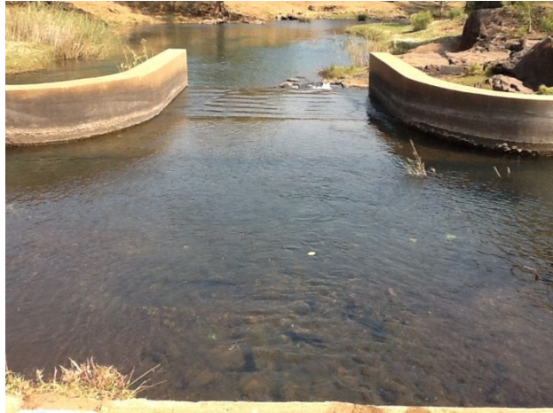
Figure 4 Department of Water Affairs weir site
